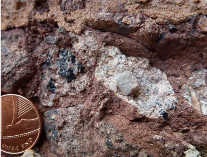
Figure 5 Granite clasts within a block of breccia in the wall of St Stephen's Church, High Street, Exeter. Image © J.D. Mather.
