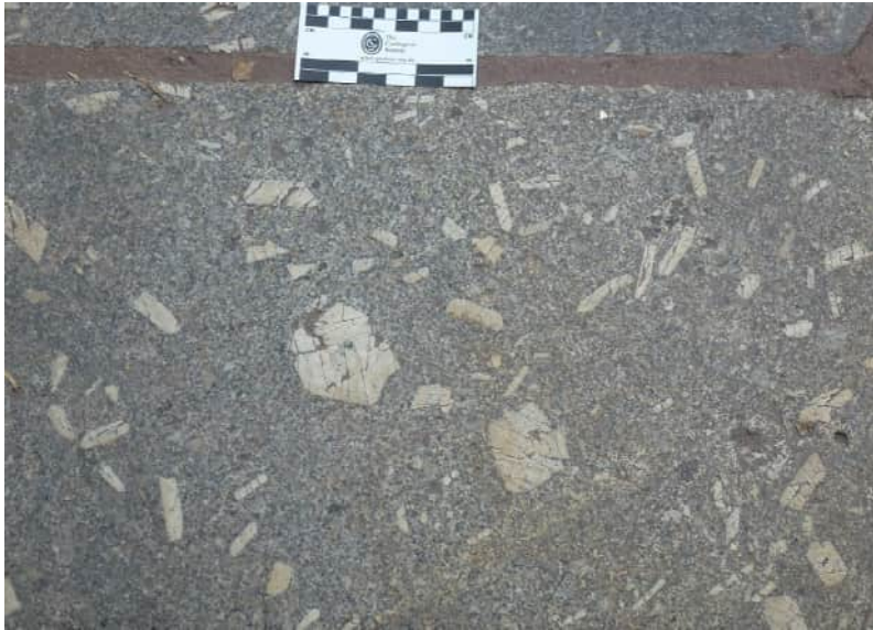
Figure 4 Pavement slabs of porphyritic granite in Cathedral Close, Exeter. Image © J.D. Mather.
